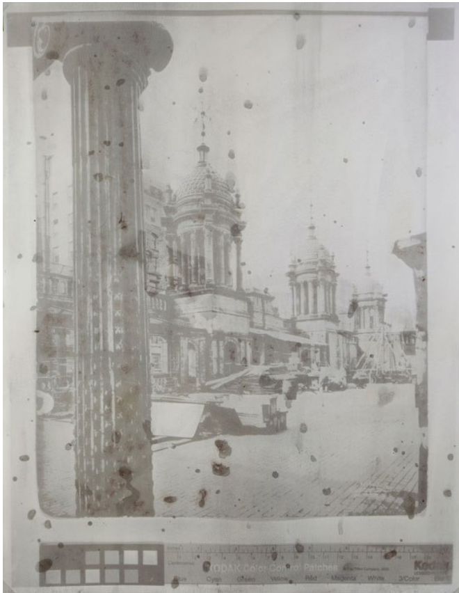
Demolition of Madison Square Garden, 1925 Matthew Brandt, 2014
