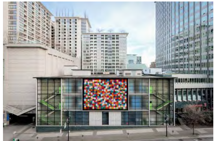
Photography star Jessica Eaton brings a shining element of vibrant newness to a fading local landmark, the Dal Grauer Substation.
