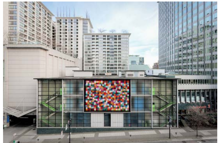
Photography star Jessica Eaton brings a shining element of vibrant newness to a fading local landmark, the Dal Grauer Substation.
