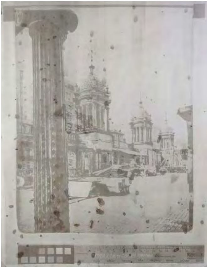
Demolition of Madison Square Garden, 1925 Matthew Brandt, 2014
