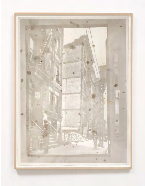
Matthew Brandt 3984846u3, Tenement row; demolition site. 1936, 2014 M+B
